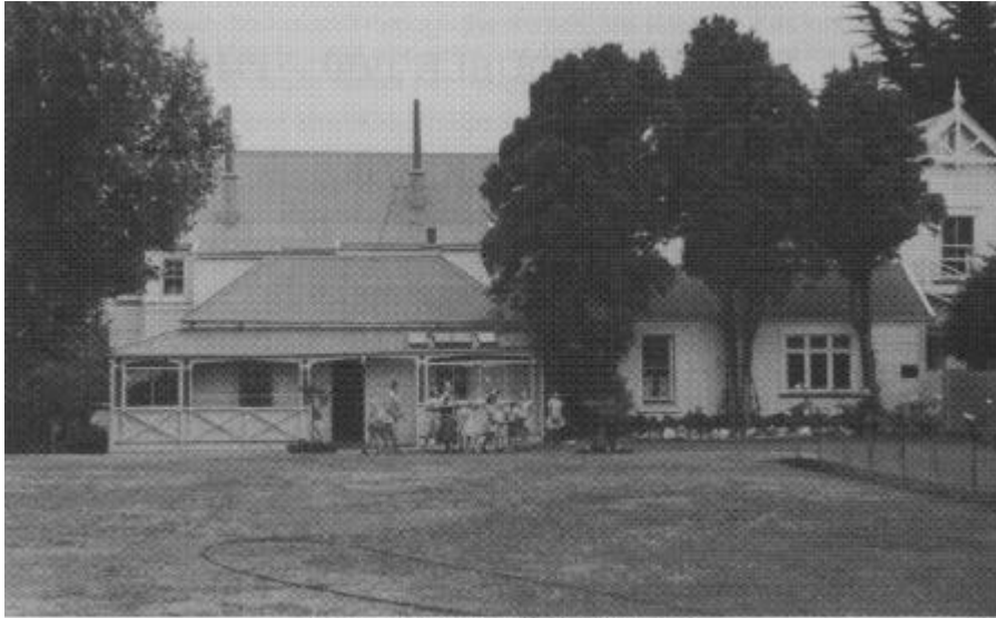
Randall House (Napier Terrace) 1955.
